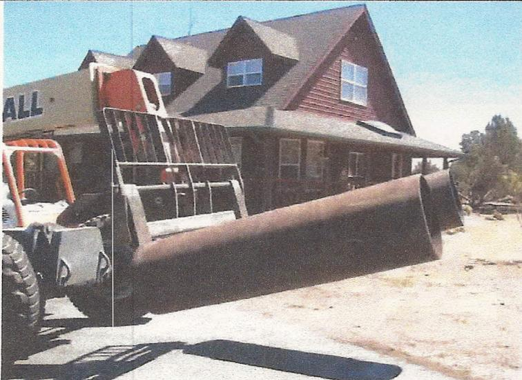
The bases for the 140' and 200' rotating monopoles are 20" OD, 19" ID Pipe 7.5' long. They will be placed in a 5' hole with rebar and concrete inside and out.
