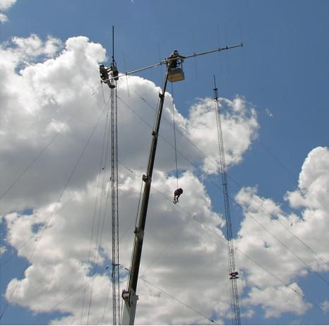
With the replacement rotator and top section in place on the 85' tower, the 7el 6M beam was installed to replace the one that blew down two years ago
