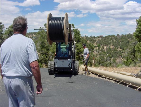
First, we had to replace old coax new 7/8" and 1/2" Heliax. W6NF and K6NV were the "pullers" for nearly 3,000' of coax and another 2,000' of replacement control cables.
