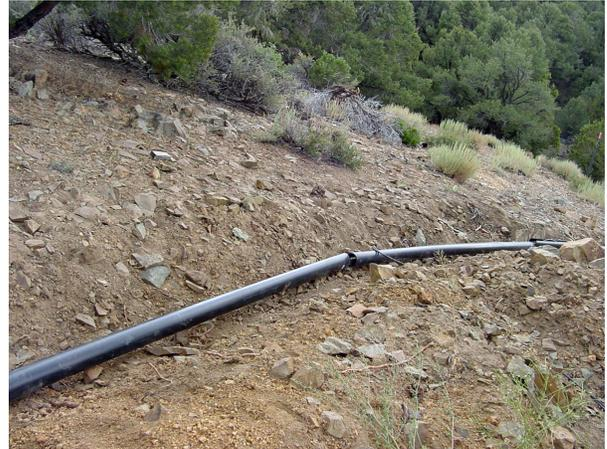
Where the ground is very rocky, the cable was laid in PVC Pipe
