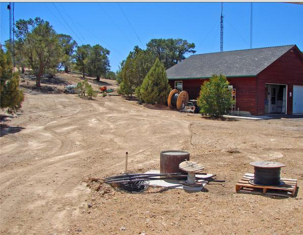
After more than a year of open trenches, the feedlines are finally buried. This is the base for the 80M Monopole (20" steel pipe in 3 yards of concrete)
