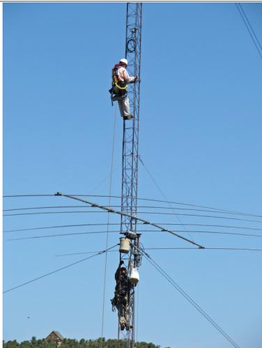
Replaced the damaged C31XR on the 20M rotating tower with a third 6 el 20
