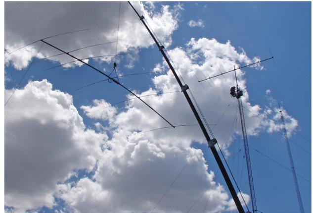
A more robust 6el OWA design 20M beam replaced the damaged 5 el F12
