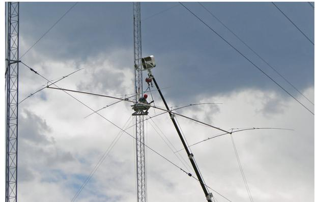
Replacing the 4el 40M beam that was taken down last summer
