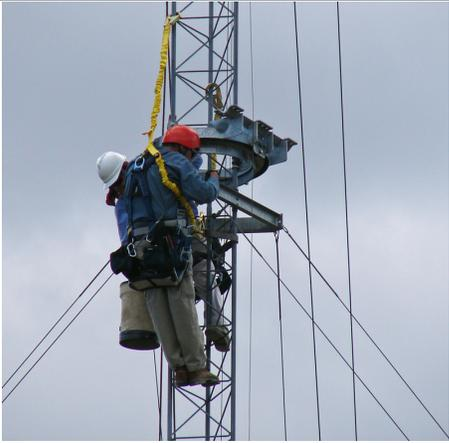
Installation of the K0XG rotating ring on the 40M tower was a chore
