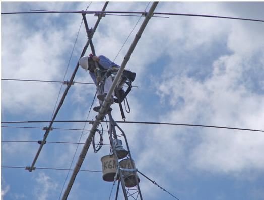
K6NA perched on the boom of the OWA 20 rigging the truss cable
