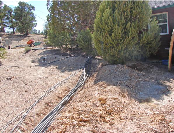
Old Cable on the Left. New Cable in the Ditch
