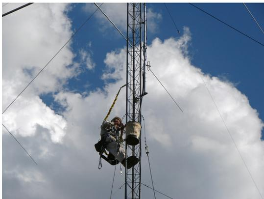
K6NA replacing damaged guy wires on the 85' Tower
